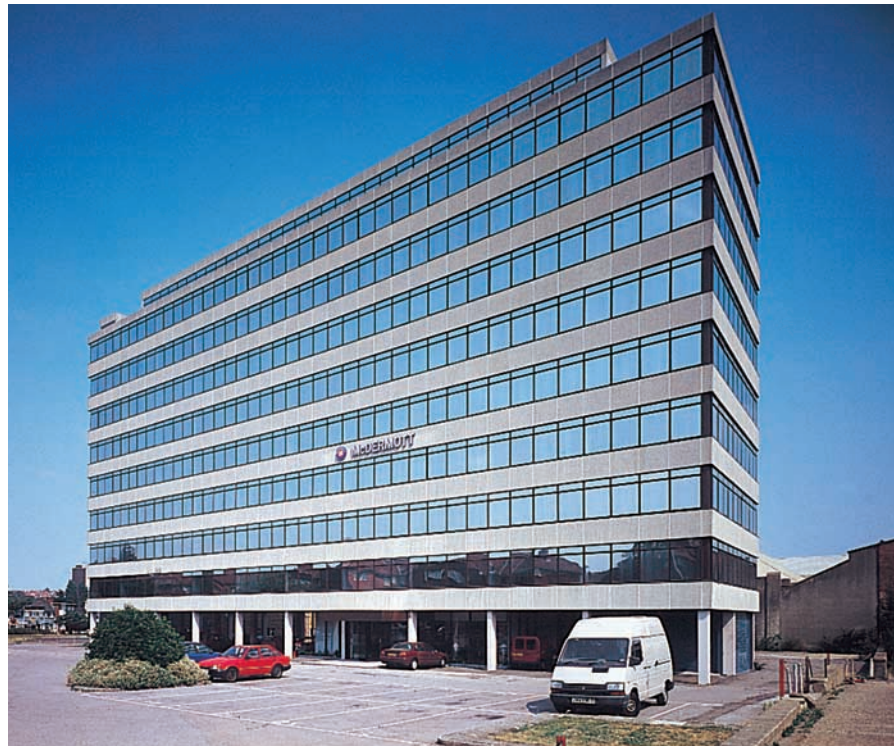
An application of silver film transforms the appearance of a 1960's office block.
